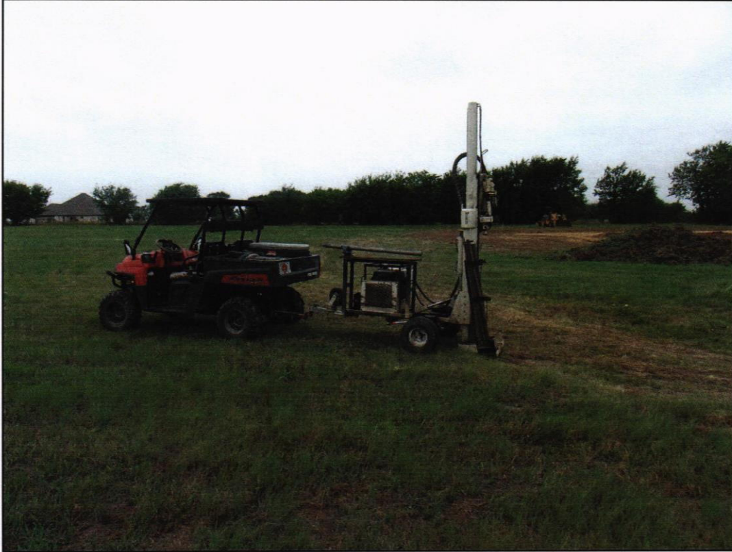
Figure 1: Picture of the Geo Probe During Soil Collection at Bore Hole 1.
